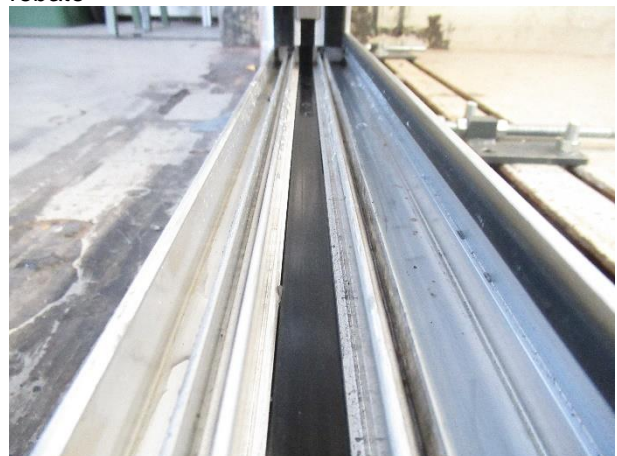
Picture 18 Seen from rebate bottom track
