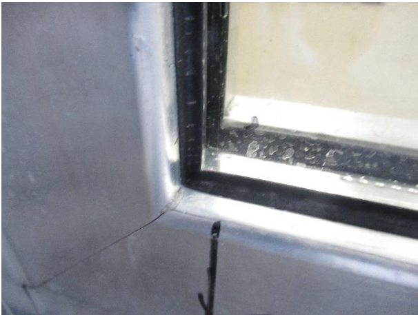
Picture 27 External glass retention
