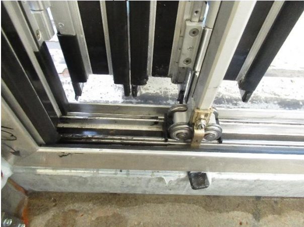
Picture 11 Fold & slide element sash open
