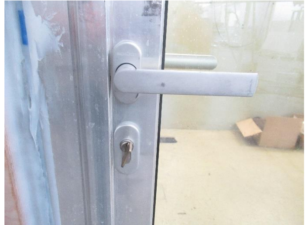
Picture 26 Lever handle, lock cylinder with rosette
