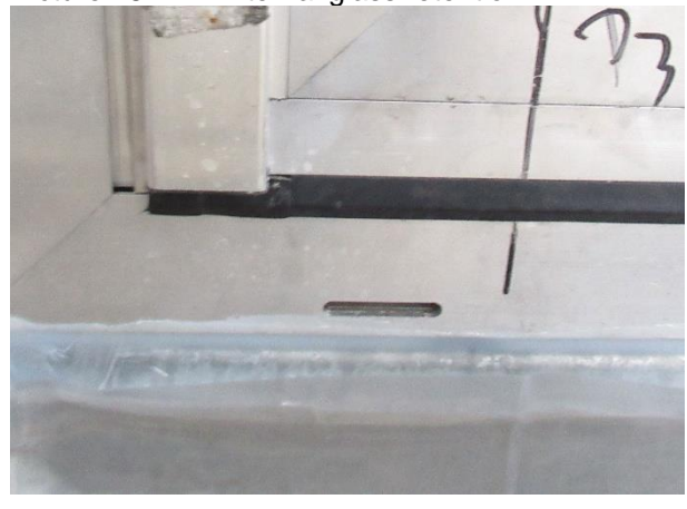
Picture 30 Drainage to outside front
