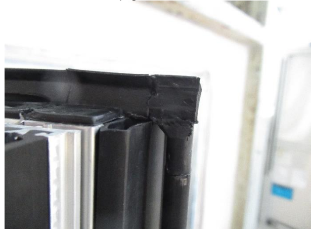
Picture 12 External rebate seal, corner design
