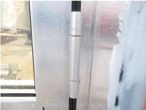
Picture 15 External door hinge inactive sash
