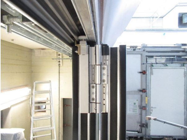
Picture 9 Top guide roller
