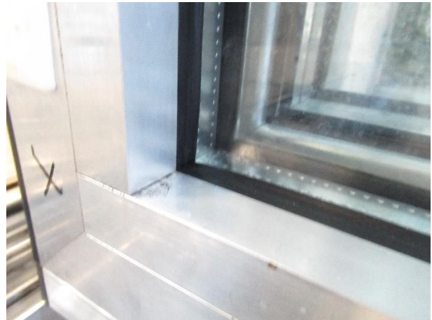
Picture 28 Internal glass retention
