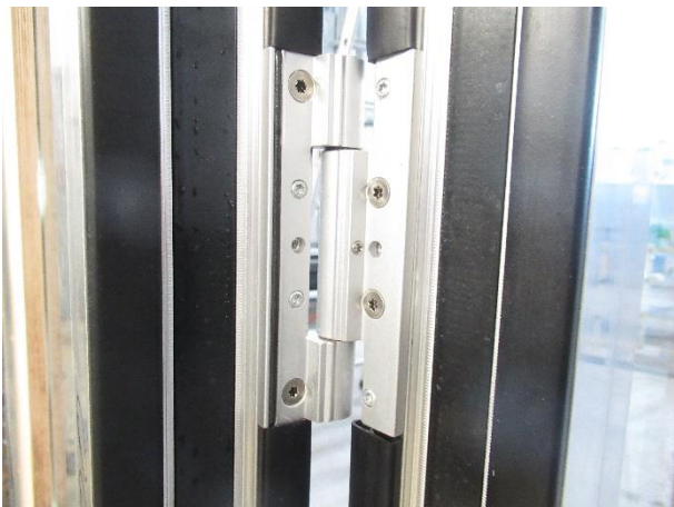
Picture 17 Door hinge inactive sash, seen from rebate
